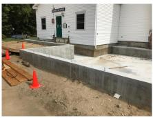
The addition of a new community room is moving along. Sometimes we have to hurry up and wait for the next stage of construction but progress is being made. The new septic system is installed, the old concrete ramp demolished, the foundation excavated and poured, and a floor built. Framing has begun and the roof trusses will arrive shortly. It's exciting to be able to see where the windows and doors will be.
